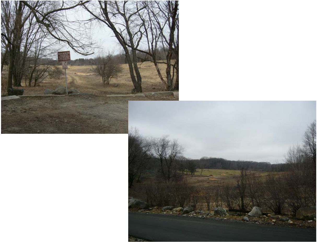
Figure 9 April 2008 Images, after restoration has begun.
